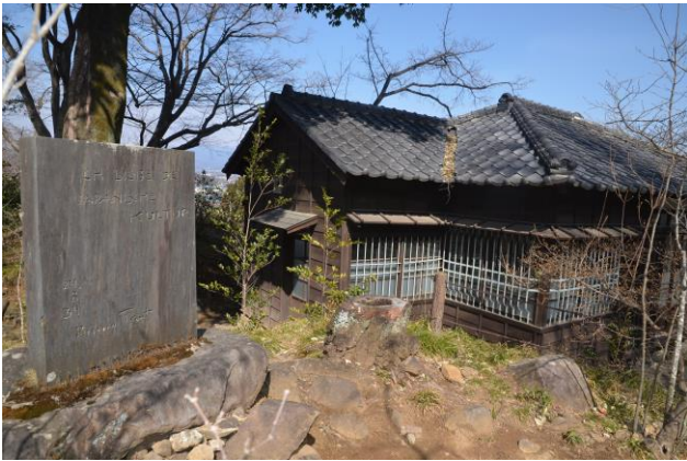
Photo 4 Outside View of Senshintei
