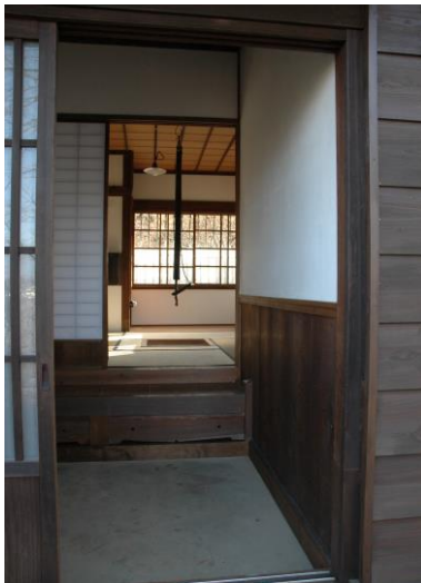
Photo 5 Inside View of Senshintei
