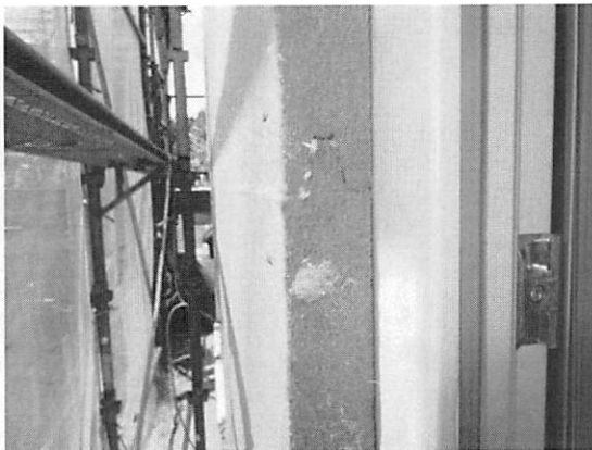
Fig.-6 ETICS using Wooden Fiber
