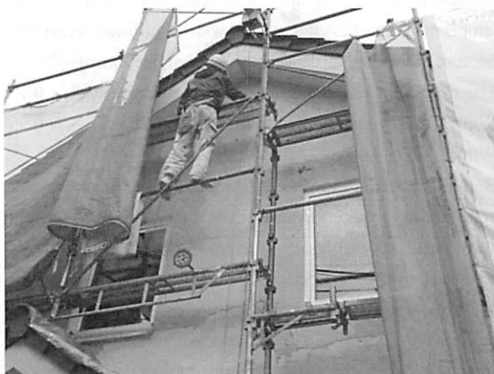
Fig. 3 Plaster work with adhesive mortar on the wooden fiber board
